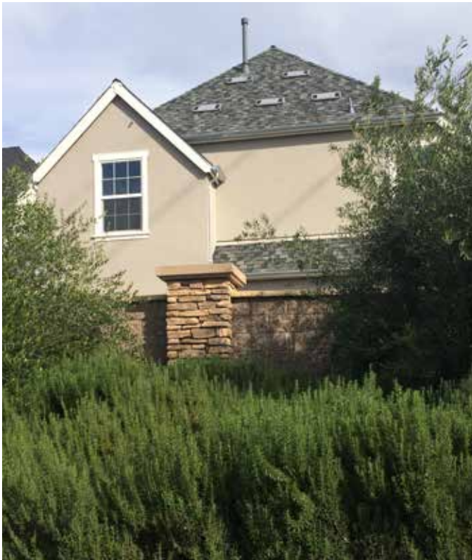
Landscaping in Front of Masonry Wall
