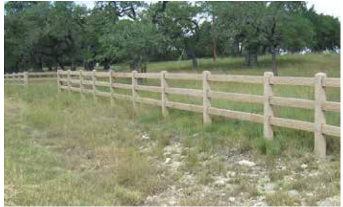
Concrete Rail Fencing
